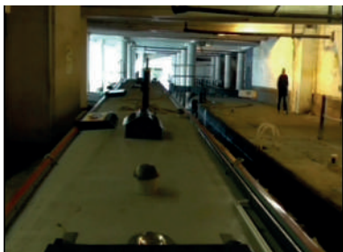
(Left) Underground lock near the top of the Rochdale
