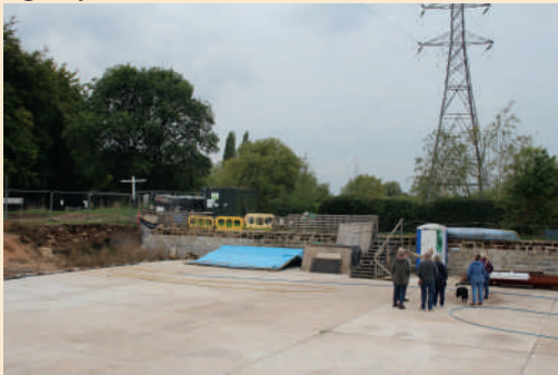
Almost all of the basin floor is now concreted. The bund will remain until the bridge is complete.
