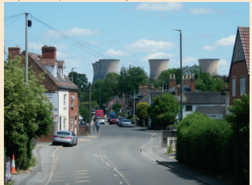
A soon to be historic view of Willington village, with the cooling towers of the now redundant power station in the background. [Steve Whetnall]
